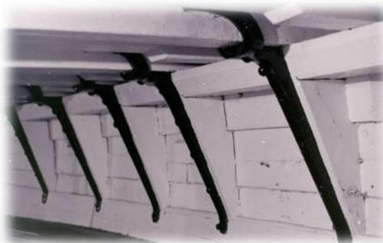
Built during the Industrial Revolution, Unicorn carries several innovative features, including iron knees and riders. These metal fixtures can be found throughout the ship and provided Unicorn with additional structural strength.
