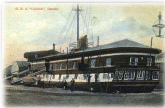
One of the most distinctive features on board Unicorn – the ship's roof – was constructed shortly after Unicorn was placed in reserve in the 1820s. It is now the only remaining example of this once common fitting.
